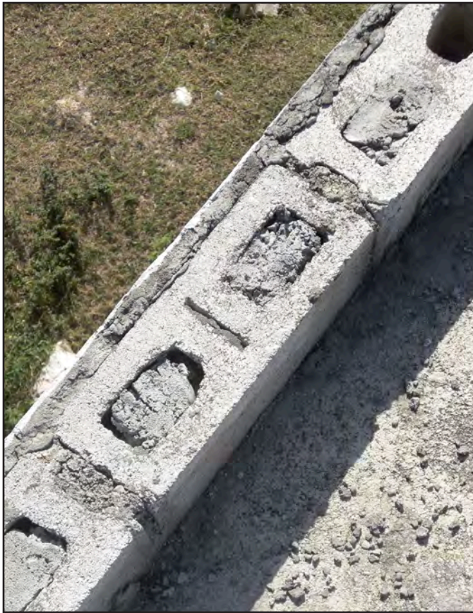
Fig. 1.53_ CMU block wall of the COTN office
