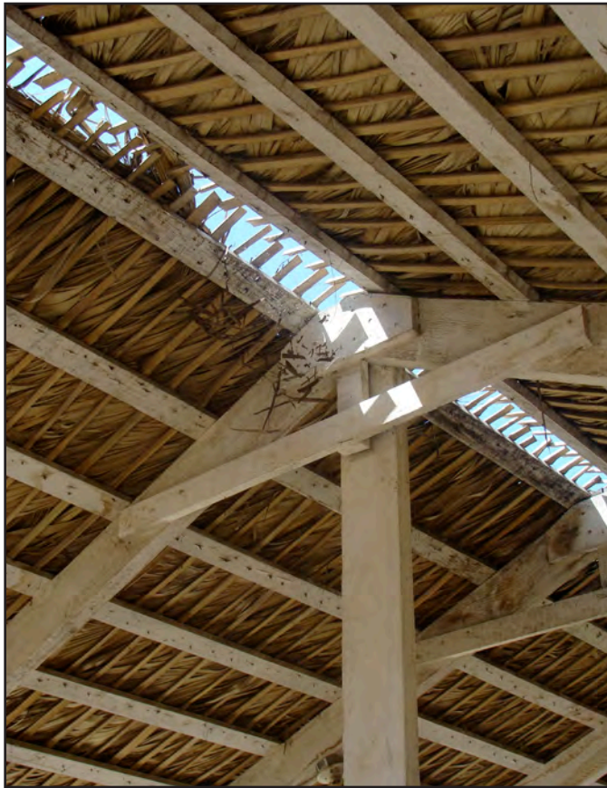
Fig. 1.51_ Roofing connection problem; school in Batey Algadon
