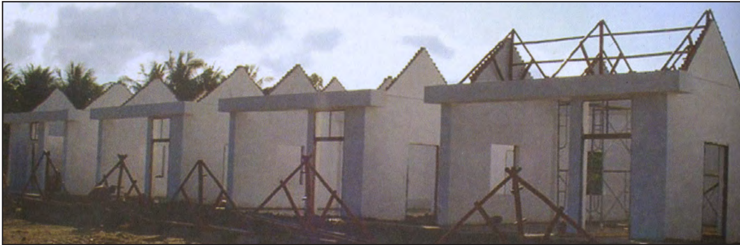
Fig. 1.66_ Construction of the classrooms in modular forms
