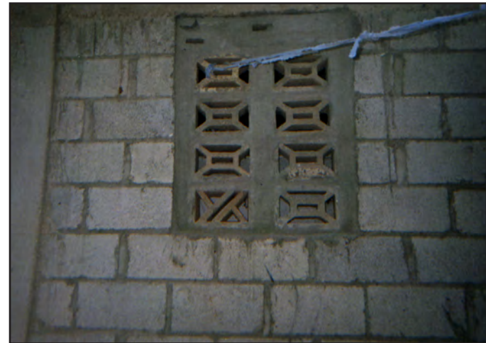
Fig. 1.10_ Concrete blocks to allow air flow
