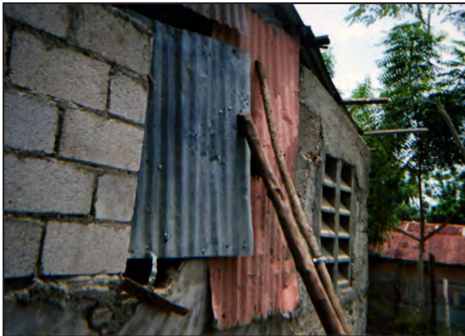
Fig. 1.17_ The exterior windows covered with metal sheathing
