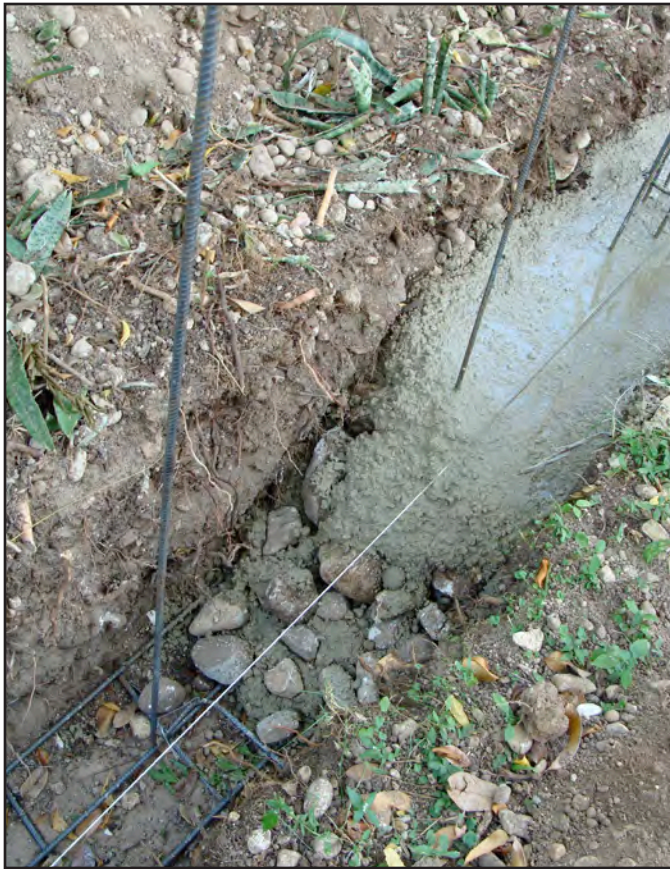
Fig. 1.57_ Use of large rocks within the foundation of the wall
