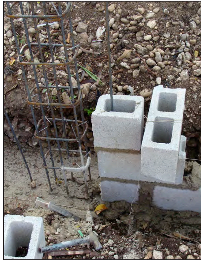
Fig. 1.56_ Detail of the use of rebar within a CMU block wall
