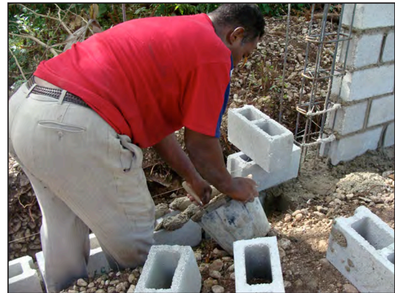
Fig. 1.58_ Building technique with CMU block
