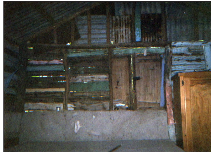
Fig. 1.12_ The house walls made up of different wooden slats
