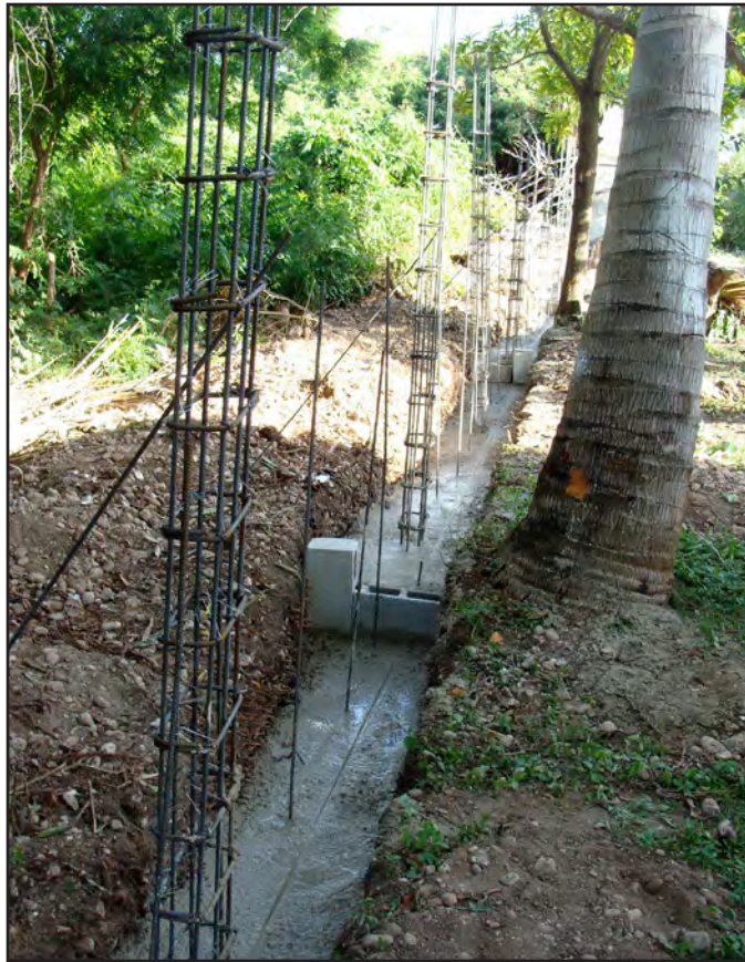
Fig. 1.55_ Foundation pouring for wall at Casa Besteda
