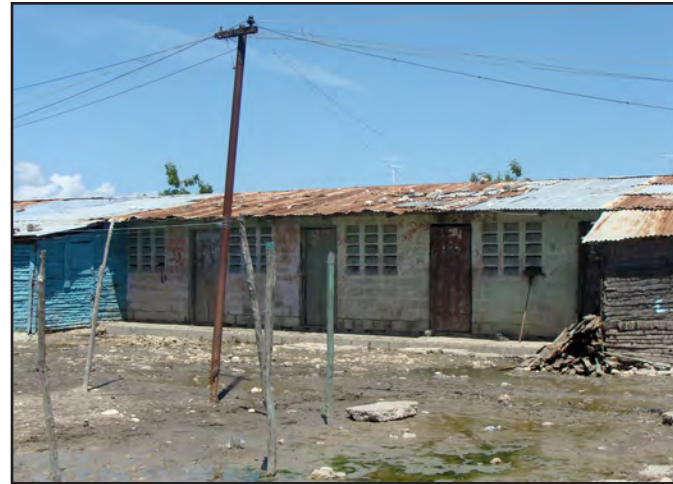
Fig. 2.5_ CMU block housing in the Batey Algodon
